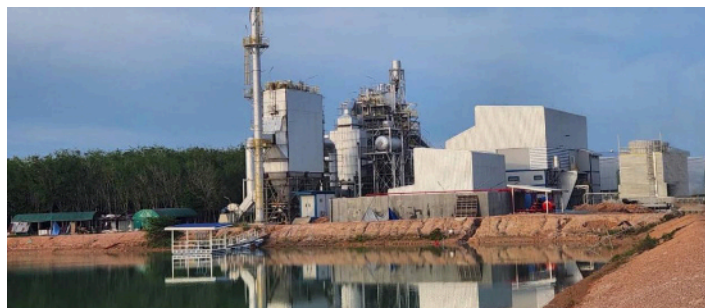
The Pracharat Biomass Mae Lan power plant in Pattani
